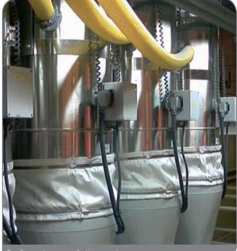
Feeding system on a plastic conveying process
